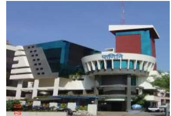
Senapati Bapat Road, Pune (operational)
