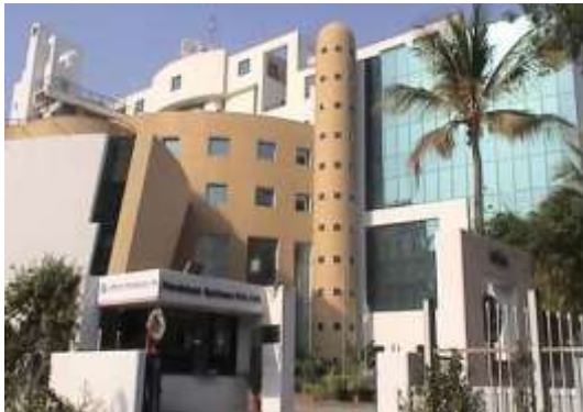
Senapati Bapat Road, Pune (operational)
