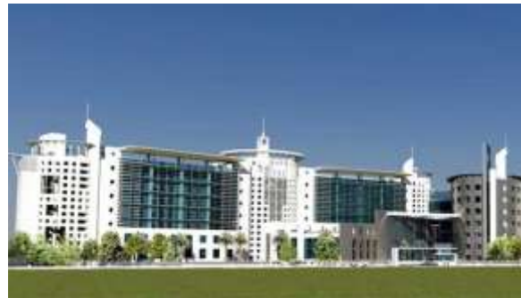
Under construction (artist impression)
